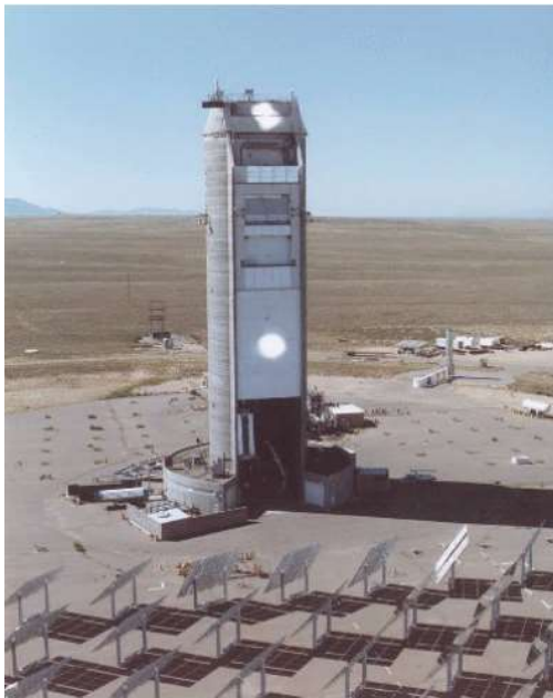
MSEE solar tower thermal power station in the United States
