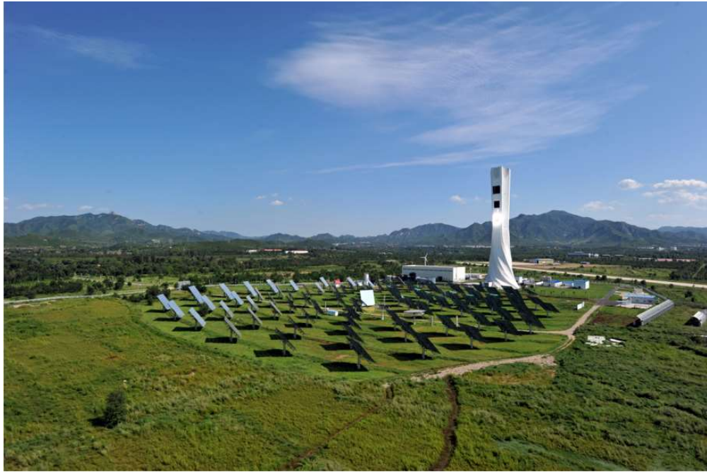
Entrapment tower of Badaling power station in Yanqing
