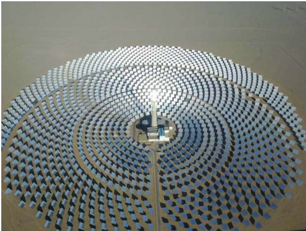
The solar tower in Dunhuang, Gansu, China
