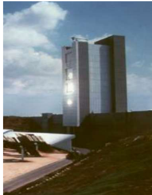
Weizman Solar Tower Thermal Power Station in Israel
