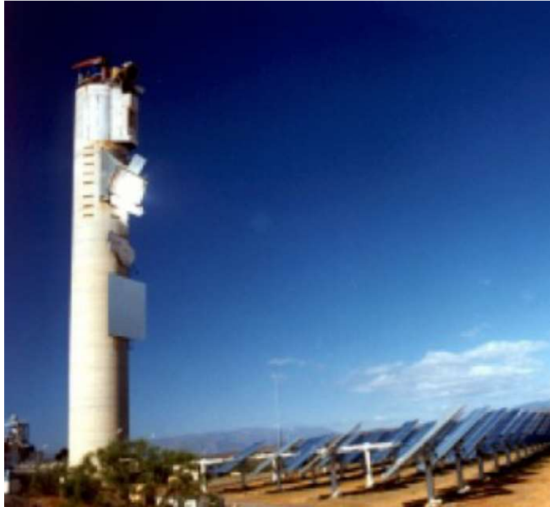
CESA-1 solar tower thermal power station and 60m high tower
