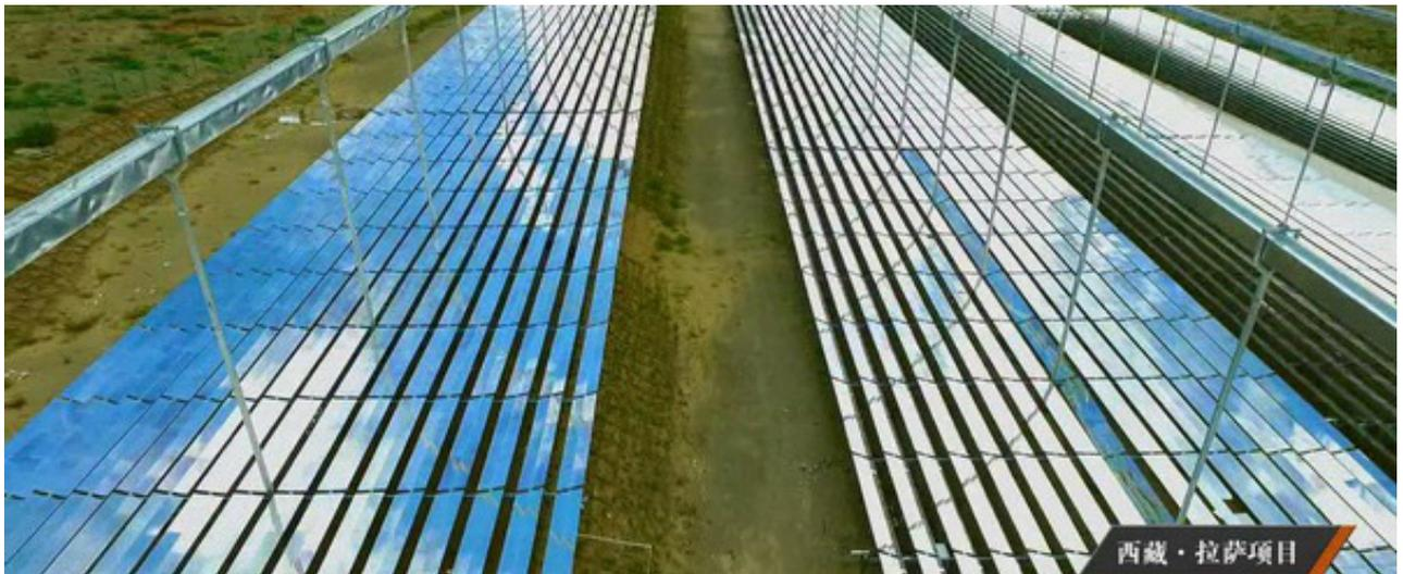
Figure: 1 MWe Linear Fresnel CSP Cogeneration Power Plant in Liuwu New District, Lhasa (Source: DCTC)
