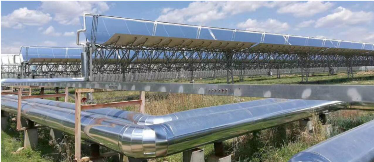
Figure: China's First 1 MW Parabolic Trough CSP Plant (Source: Institute of Electrical Engineering, Chinese Academy of Sciences)
